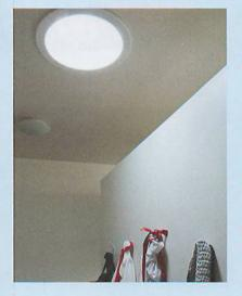
light then travels through highly reflective tubes and is diffused into the rooms via dual-glazed acrylic lenses in the ceilings. The materials used to make the tubes prevent heat gain and loss and UV transmission. From inside the house, the lenses resemble average light fixtures. They even have optional built-in dimmers for when the daylight is too intense and optional electric bulbs that can be flipped on at night.
